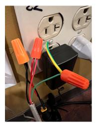
The Springtree WallDim1 and Wall-Dim5 should be grounded in order to prevent static shock damage. Using a short 18 gauge whip the WallDim units can be grounded to the outlet that is providing power.
